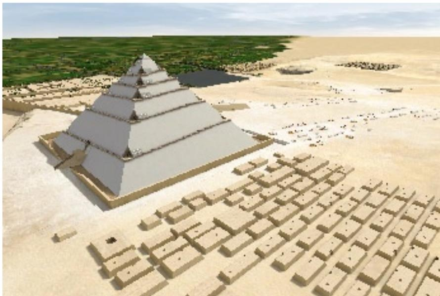
Twentieth year of the reign. The summit is reached. Finishing work is about to start descending from the summit: the recesses are being filled in, the outside gangway is being dismantled, the last roughly cut facing blocks are being surfaced.
