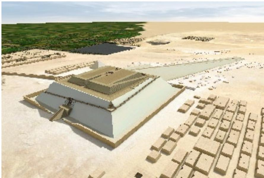
Fifteenth year of the reign. The site is at levels +43 m and +54 m, seen from the North West. All the rafters of the King's Chamber are now located within the pyramid, either in the storage area on level +43 m or already in place in the first 3 ceilings. The external ramp is still in service and supplies the materials being used to construct the second degree.
