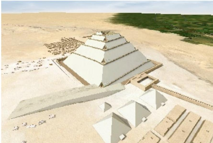
Nineteenth year of the reign. The construction, seen from the North West, has reached level +113 m. The King's Chamber has been finished for some time. The pyramid is being constructed with the materials recovered from the demolition of the external ramp. The blocks are now transported to their final positions via the internal ramp.
