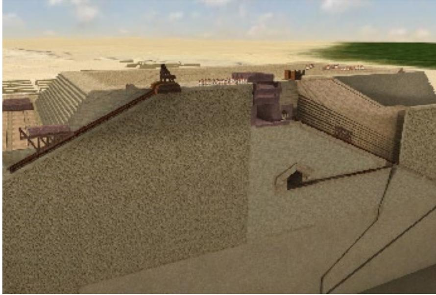
Fifteenth year of the reign. The granite rafters that form the King's Chamber are raised by means of the counterweight and positioned definitively in each of the ceilings. Floor by floor, the King's Chamber is constructed with the help of the counterweight, which considerably reduces the number of workers required.
