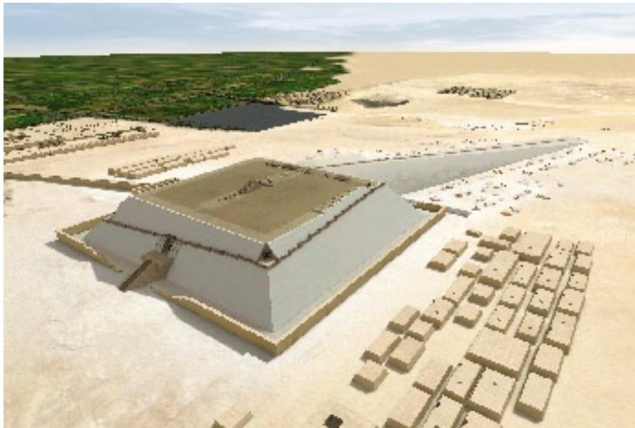
Fourteenth year of the reign. Construction of the site has reached the +43 m level, as seen from the North West. The external ramp has reached its maximum level. The interior ramp already has three flights but because of its geometry, it does not affect supply to the site. The ceiling rafters of the King's Chamber are raised to this level by means of the counterweight operating in the Great Gallery.
