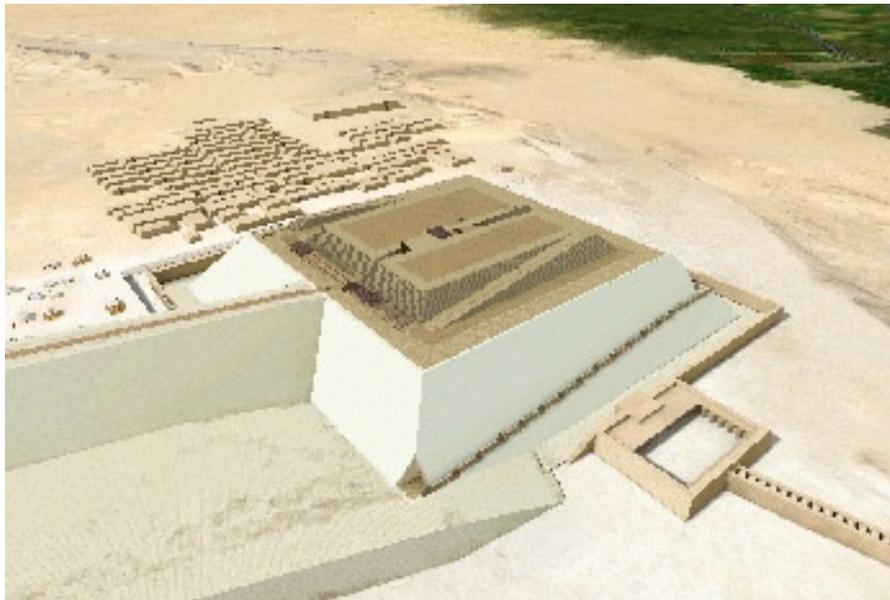
Fifteenth year of the reign, the pyramid looks like a two degree pyramid: the first degree, which is definitive, from the base to level +43 m, The second degree stands some twenty metres back from the faces, from level +43 m to level +54 m. This degree is built around the King's Chamber as the chamber is constructed. At level +54 m, the third ceiling is being put into place.
